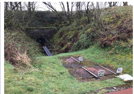
There are two raw water sources that serve Prewley WTW – the new raw water transfer main to Northcombe WTW will diversify the source water available at Northcombe WTW which currently only has Roadford water available. This image shows the end of the existing gravity abstraction into Prewley WTW from Vellake.
