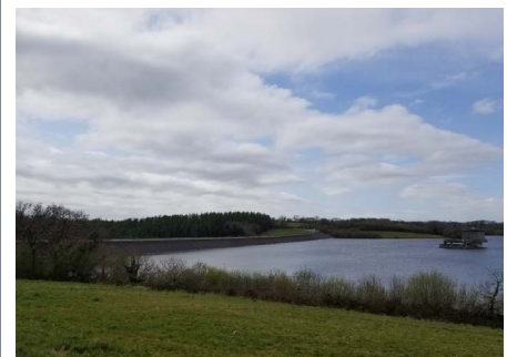
The Roadford Pumped Storage scheme will increase the resilience of the regional water supply system by enabling Roadford Lake to be topped-up during winter months.
