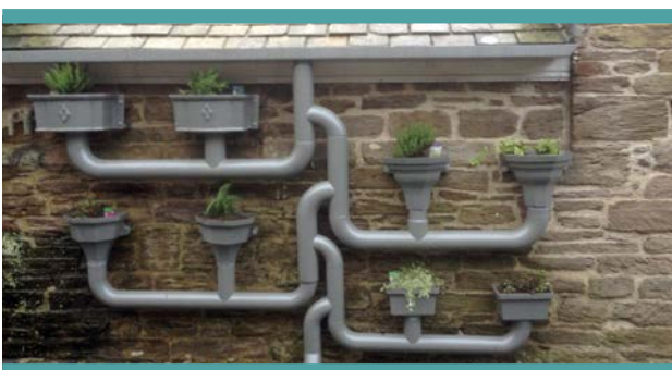
Photograph: Flow mitigation installation, Aveton Gifford
