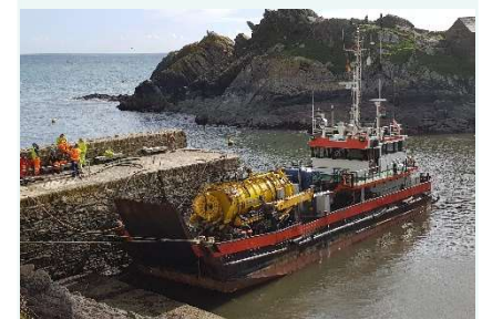
Top: Sidmouth Beach Centre: Reed Bed Bottom: Polperro Sewer Jetting
