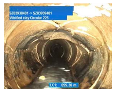
Collapsed pipe
