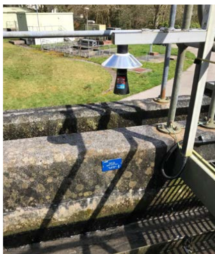
EDM ultrasonic head
