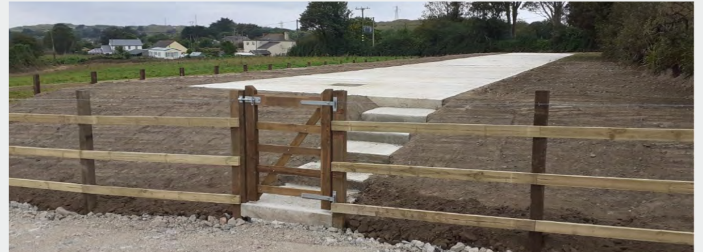
The finished site
