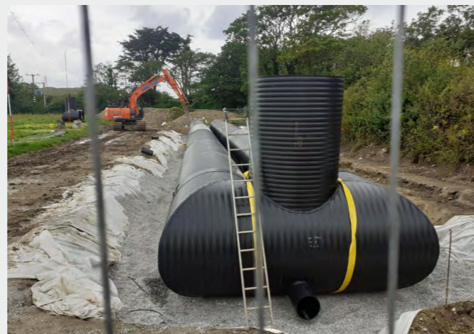
Weholite Tank being installed
