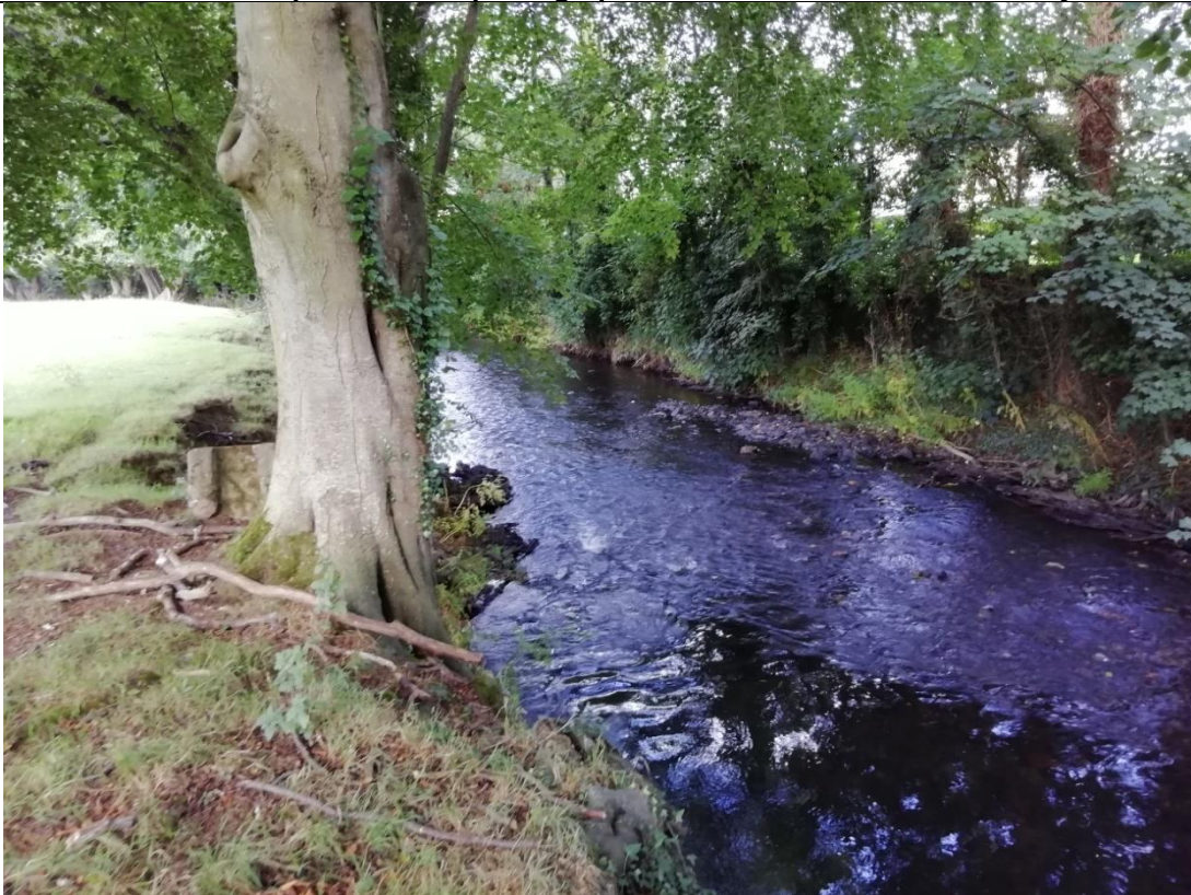
Reach L1: view downstream showing steep, undercut banks and overhanging trees with minimal sediment storage.
