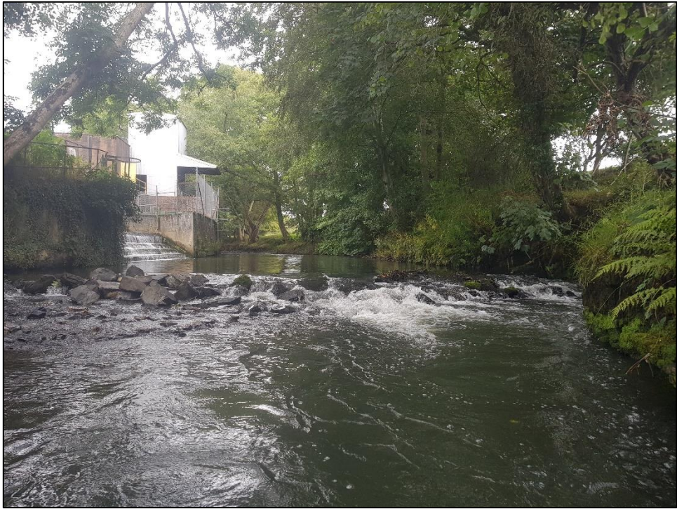
Figure 5-14 Rubble weir – River Lyd d/s Ambrosia Creamery discharge point
