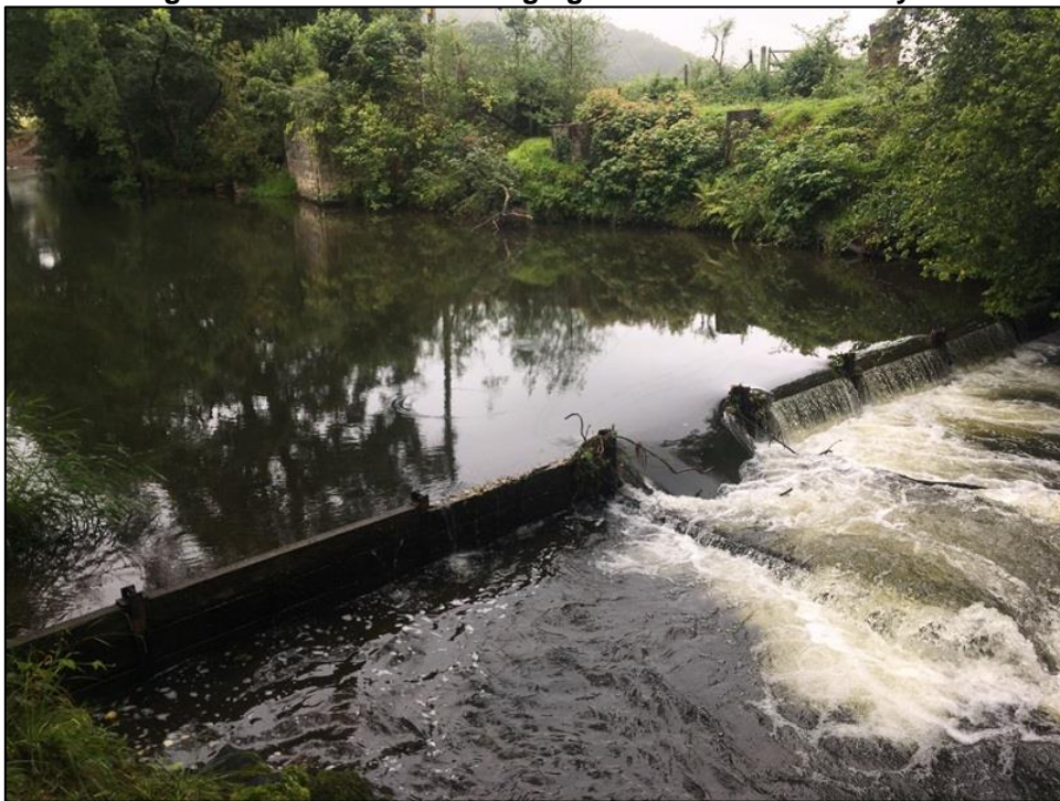
Figure 5-16 Impounding structure on the lower reaches of the River Lyd
