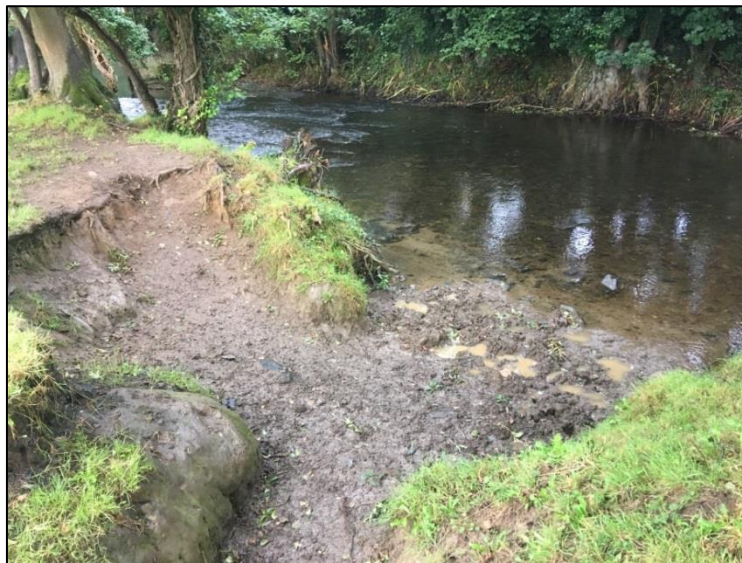
Figure 6-14 Bank erosion exacerbated by cattle poaching
