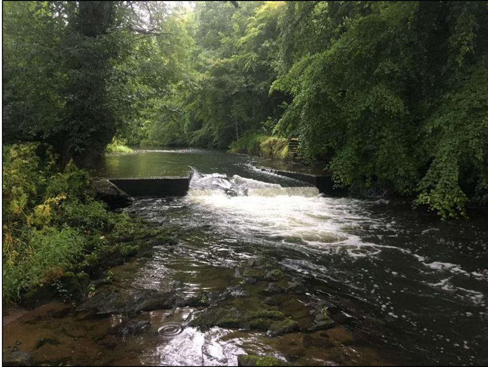
Figure 5-15 Lifton Park Gauging Station on the River Lyd
