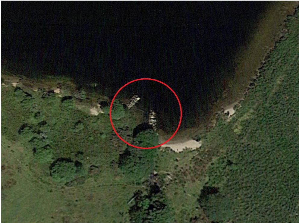
Figure 4.1: The high-level lake overflow channel (red circle), located on the southern bank of the pit. This overflow channel connects directly into the Warleggan River further downstream. Image adapted from Google Earth.
