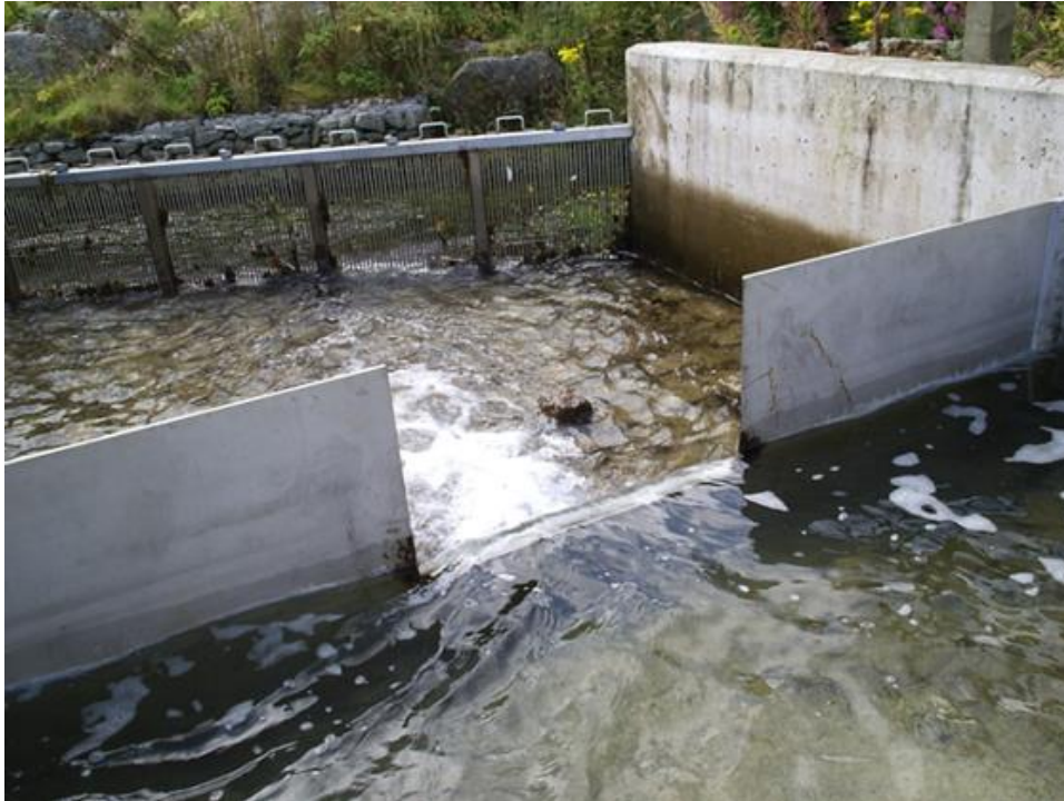
Figure 5 – Photograph of outfall screen at Park Lake
