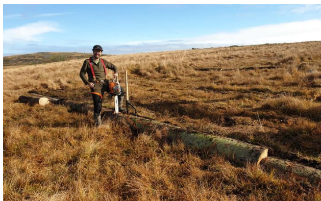
Close up of timber rounds being installed
