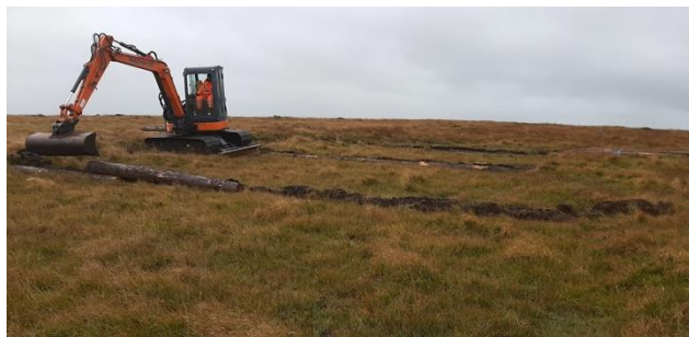
Timber rounds/logs being installed across a peat cutting
