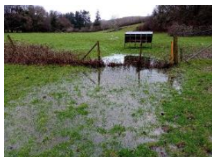
Consolidated, waterlogged soil in floodplain in the Mardle Catchment. This land has been identified as suitable for reduction in grazing intensity as well as tree-planting.
