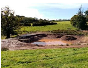
One of a series of ponds installed at Parkhouse Stream, Stoodleigh
