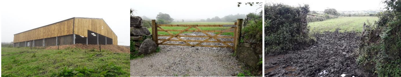
Improvements to reduce run-off
