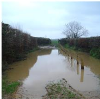
Area proposed by WRT for water diversion from farm track – Upper Tamar
