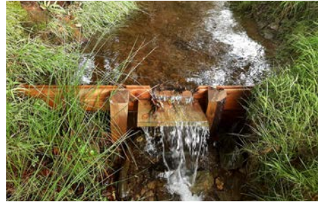
Wooden block within a boundary ditch that slows the flow of water, sediment and creates a seasonal wetland habitat
